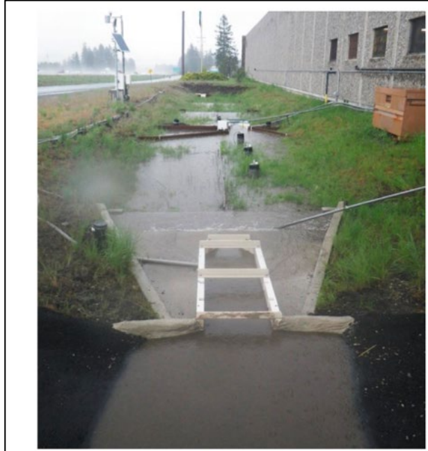
Figure 4. Example of a compost-amended biofiltration swale. Stormwater is filtered as it flows along the grass in the swale and infiltrates into the topsoil and compost. Photo: Washington State Department of Transportation.
