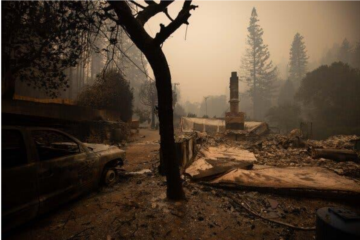
The remains of a home were surrounded by smoke after it was destroyed by the Bear Fire in Berry Creek, Calif. Photo by Christian Monterrosa for The New York Times.
